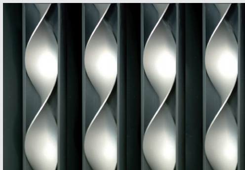
Automatic cleaning of the heat exchanger
