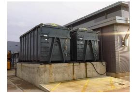
On delivery the empty bin is moved away and the full bin connected to the fuel handling system on site. Ideally one site will need at least two bins to give a continuous supply of wood chip.
