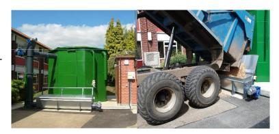
The maximum vertical lift can be up to 7 metres and the delivery speed can be between 30-50m3/hr, depending on both the chip and trough specification. The hopper is also suitable for pellets and so would allow pneumatic delivery.
